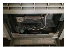
After the pilot light has been lit by the Gas Company, push in and turn the knob labeled 1-5 or 1-10 to the halfway point.
