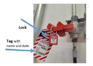
**CAUTION** – Although on/off switches, emergency 'e-stop' buttons, computer boards, and safety interlocks are safety features, they are **NOT** energy isolating devices. They can easily be turned on and off and they do not prevent accidental start-up. These safety features should never be used in place of a LOTO program.
