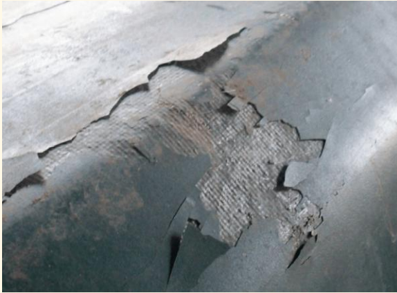
Delamination
