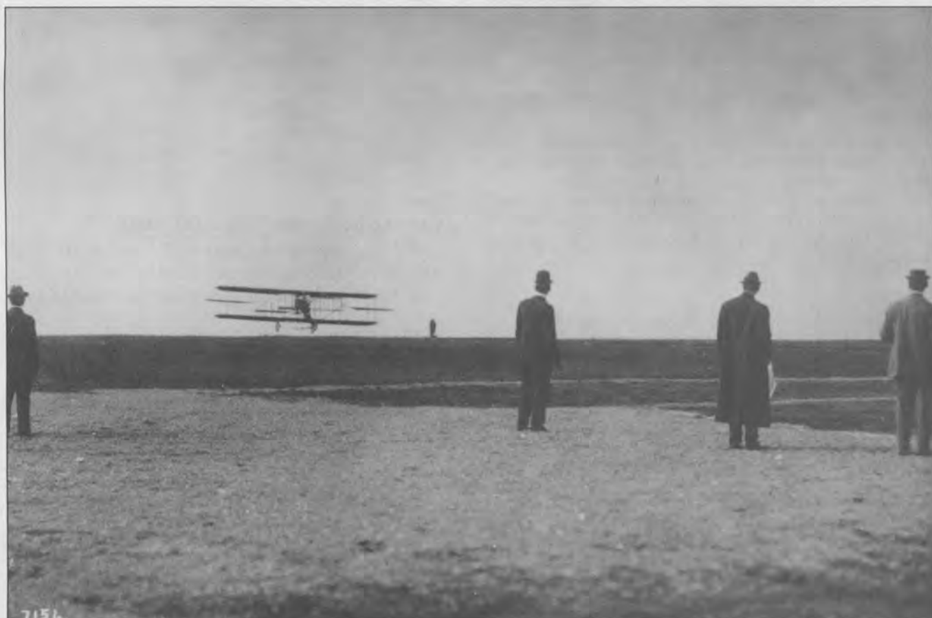
Charles F. Willard is moments from landing the "Golden Flyer" of the Aeronautical Society of New York. The four-cylinder, 22-25 horsepower Curtiss biplane was the first built by Glen Curtiss .
